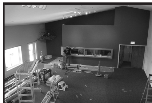
Taken May 16, 2016 - Carpet installed, room is painted, tank wall framed and painted.
